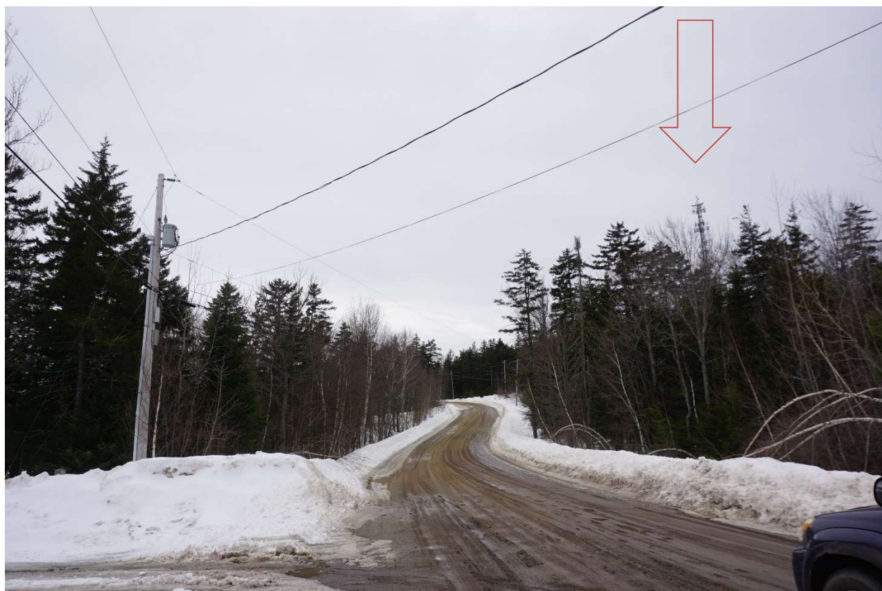
169 Oak Hill Driveway to left, the 275' cell tower can be seen on the right.
