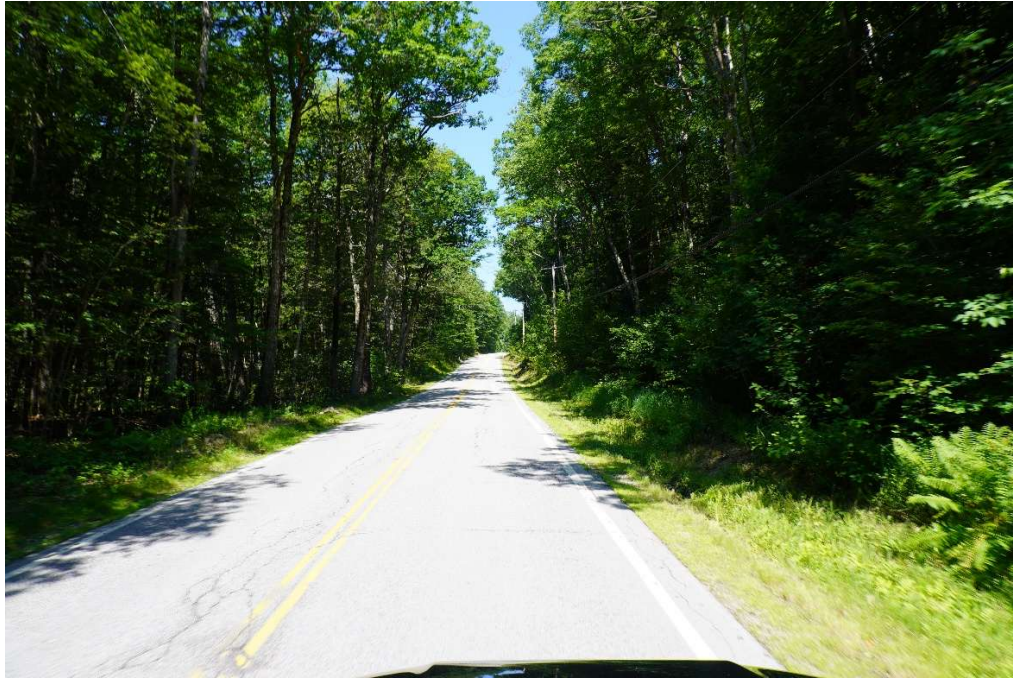
NH Route 123 – Stoddard Rd. Looking southeast
